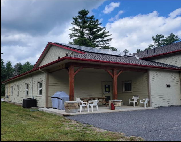
Rear of Fire Station, note solar panels on the roof
