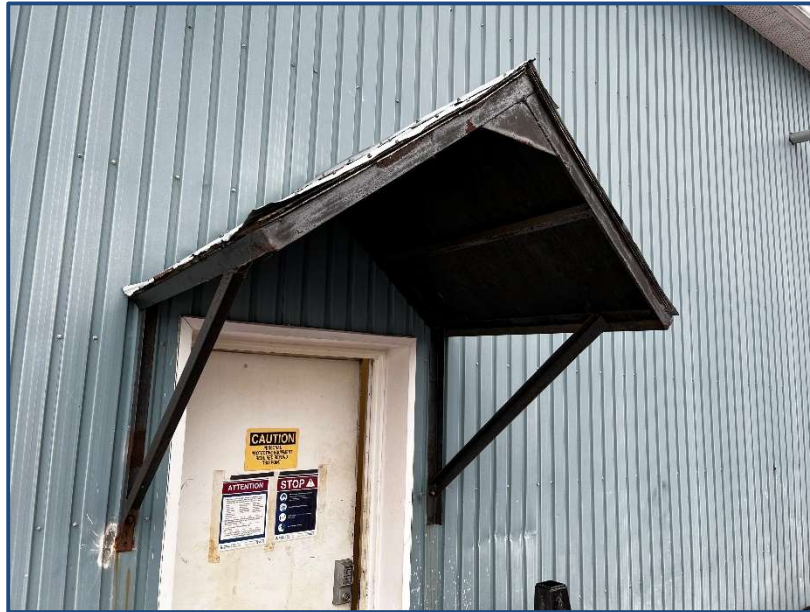
Picture 73: Garage No. 1 North Exit Opening Inwards
