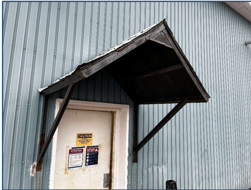
Picture 9: North Garage Side Entrance Canopy
