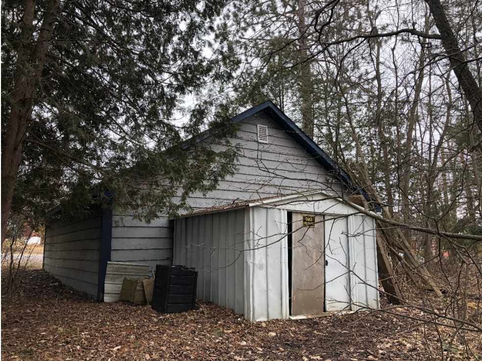
Photo 5 – Existing detached garage looking East.
