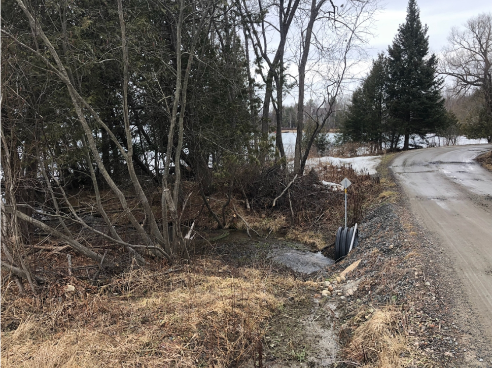
Photo #7: View of Culvert at Springfield Road.
