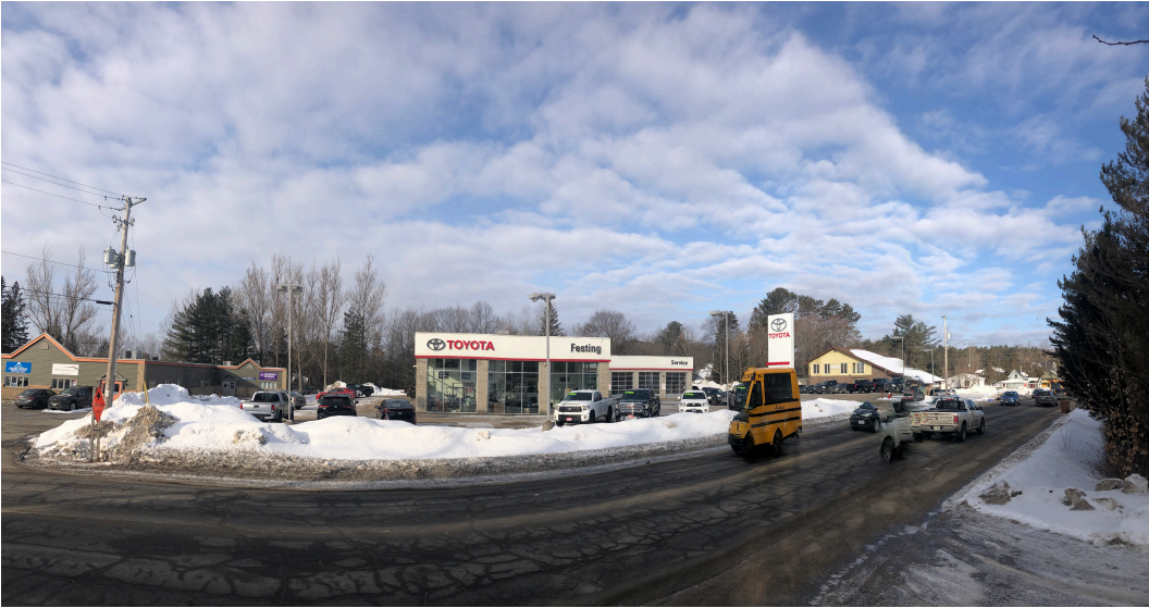
Photo #11: View of building to be expanded from Centre Street North.
